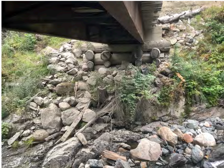
Right Bank Abutment when facing downstream
