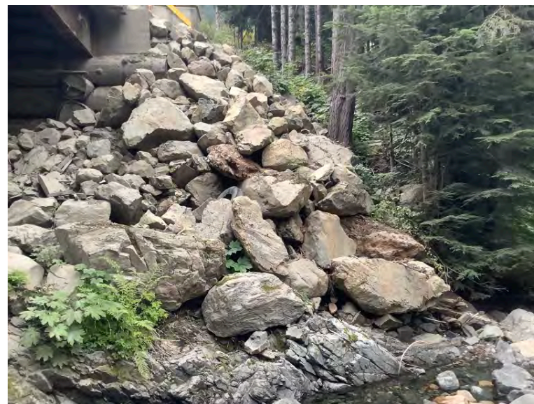
Downstream left fill slope repair
