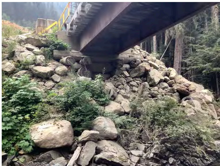
Left Bank Abutment when facing downstream
