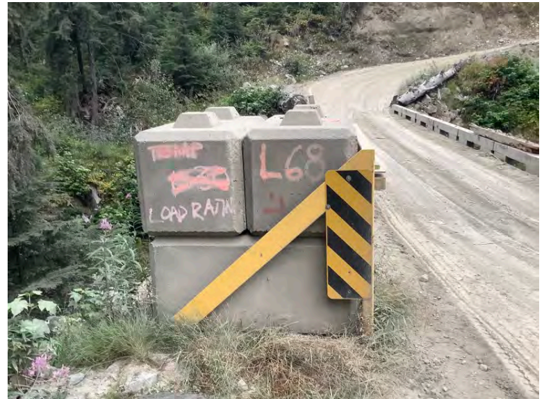
Load Rating Painted on lock block
